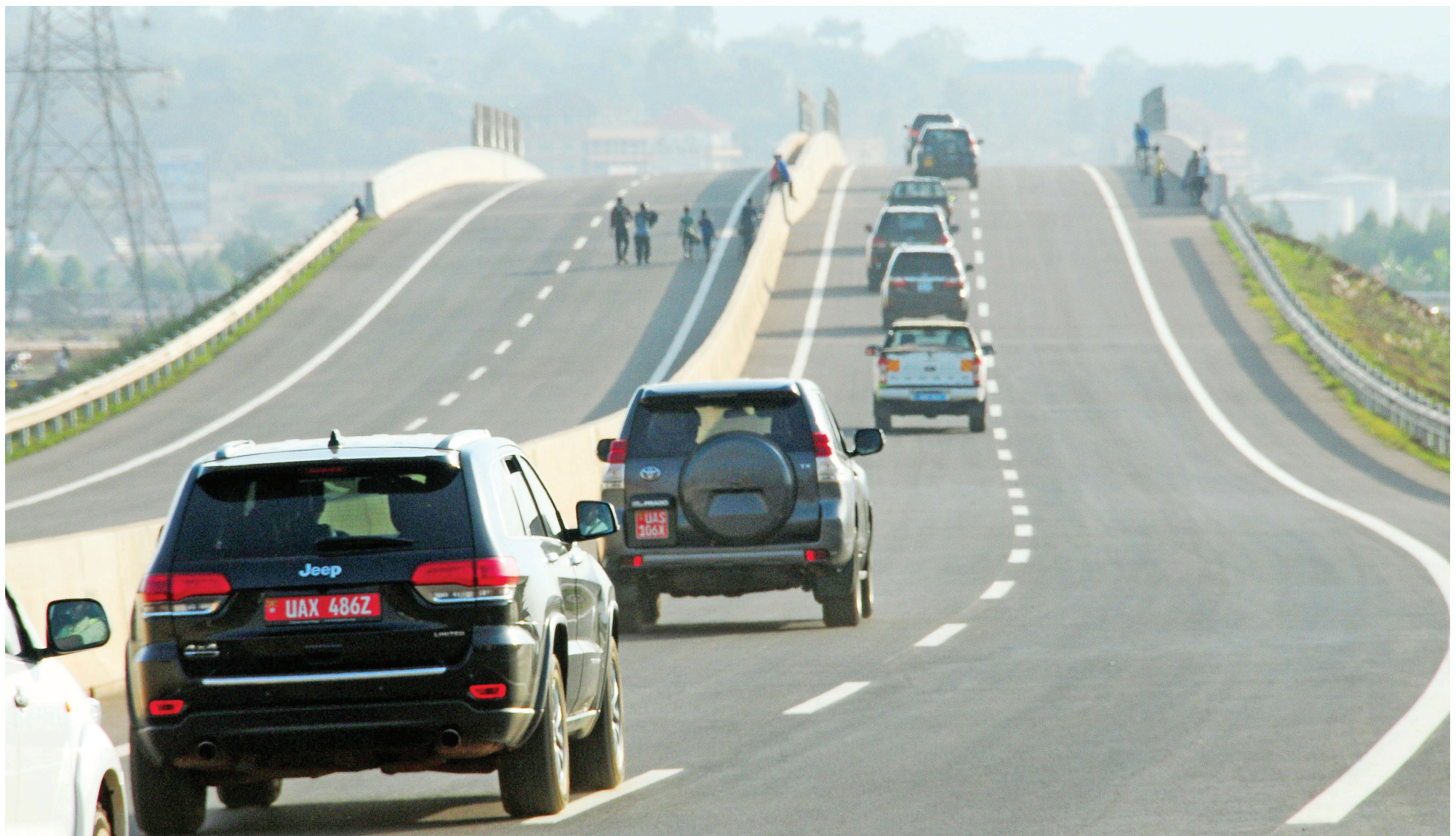
Vehicles on the the Entebbe Expressway, which was one of the most expensive infrastructure projects in Uganda. The report called for transparency on such projects
