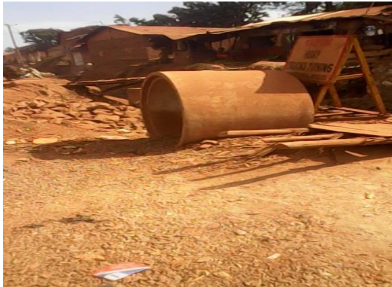
Photograph 6: Heaps of debris and culvert left on site in Namasuba Village, Makindye-Sabagabo -Wakiso District
