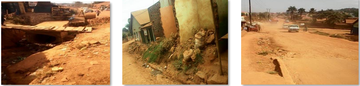
Photograph 1: From left to right; a temporary wooden bridge improvised to create access to a road-side shop in Makindye-Sabagabo, a demolished building along Najanankumbi Kikajjo Road and dusty section of Ndejje Kitiko Road.
