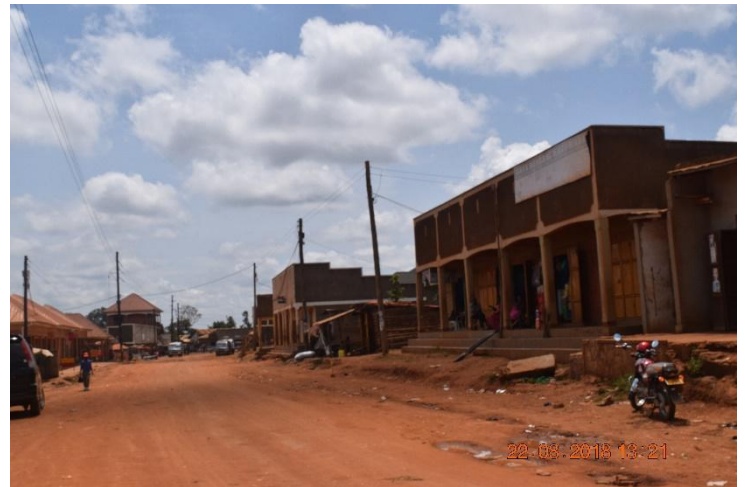
Road ready for next construction phase
