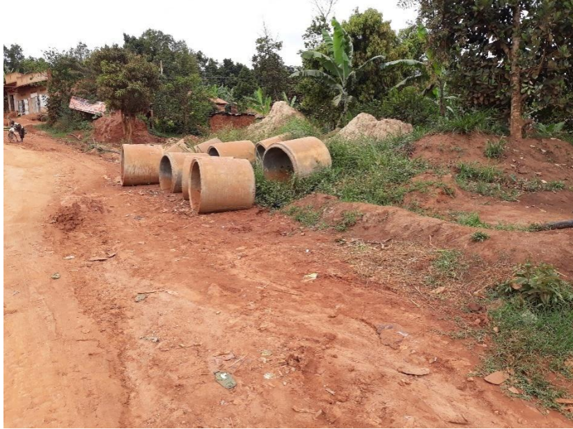
Figure8: Culverts laid along road
